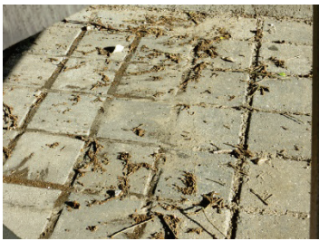
185 Sediment (poor)
