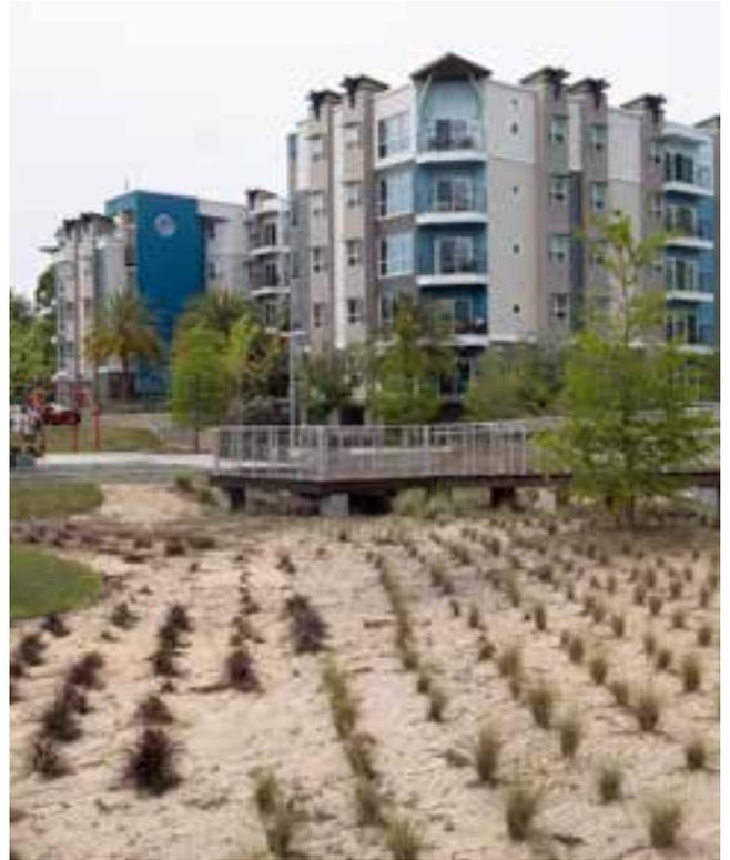
**Figure 11.** New plant installation in infiltration basin.
