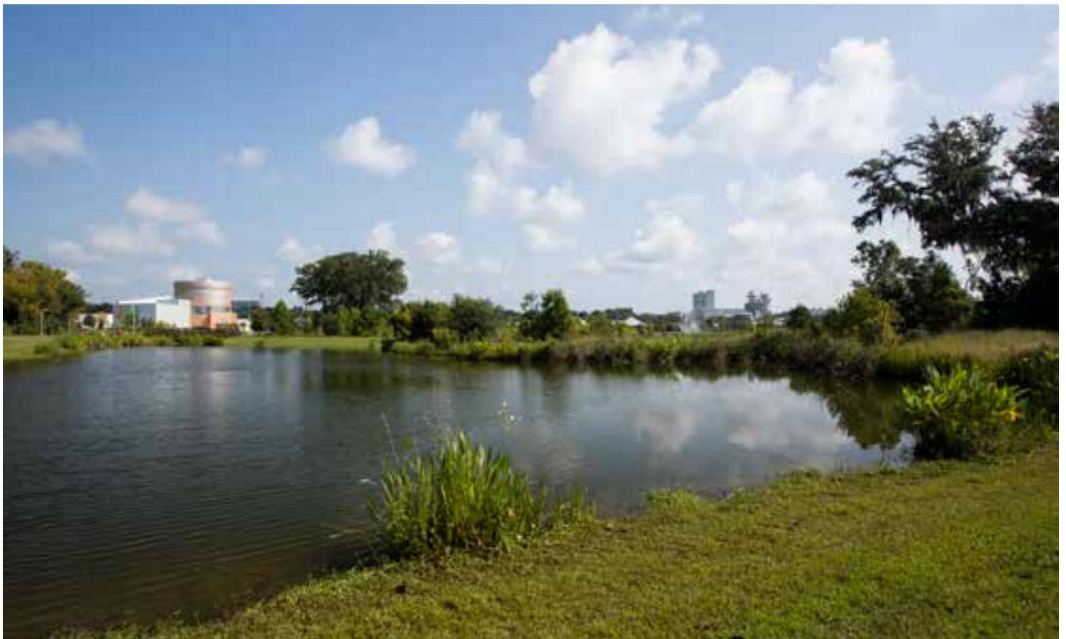
Figure 12. Stormwater pond with planted edge in Gainesville, FL.
