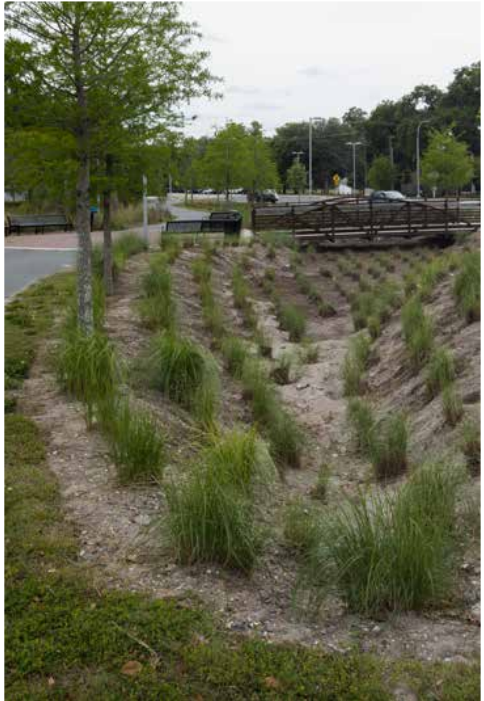
Figure 7. Bioswale in Gainesville, FL
