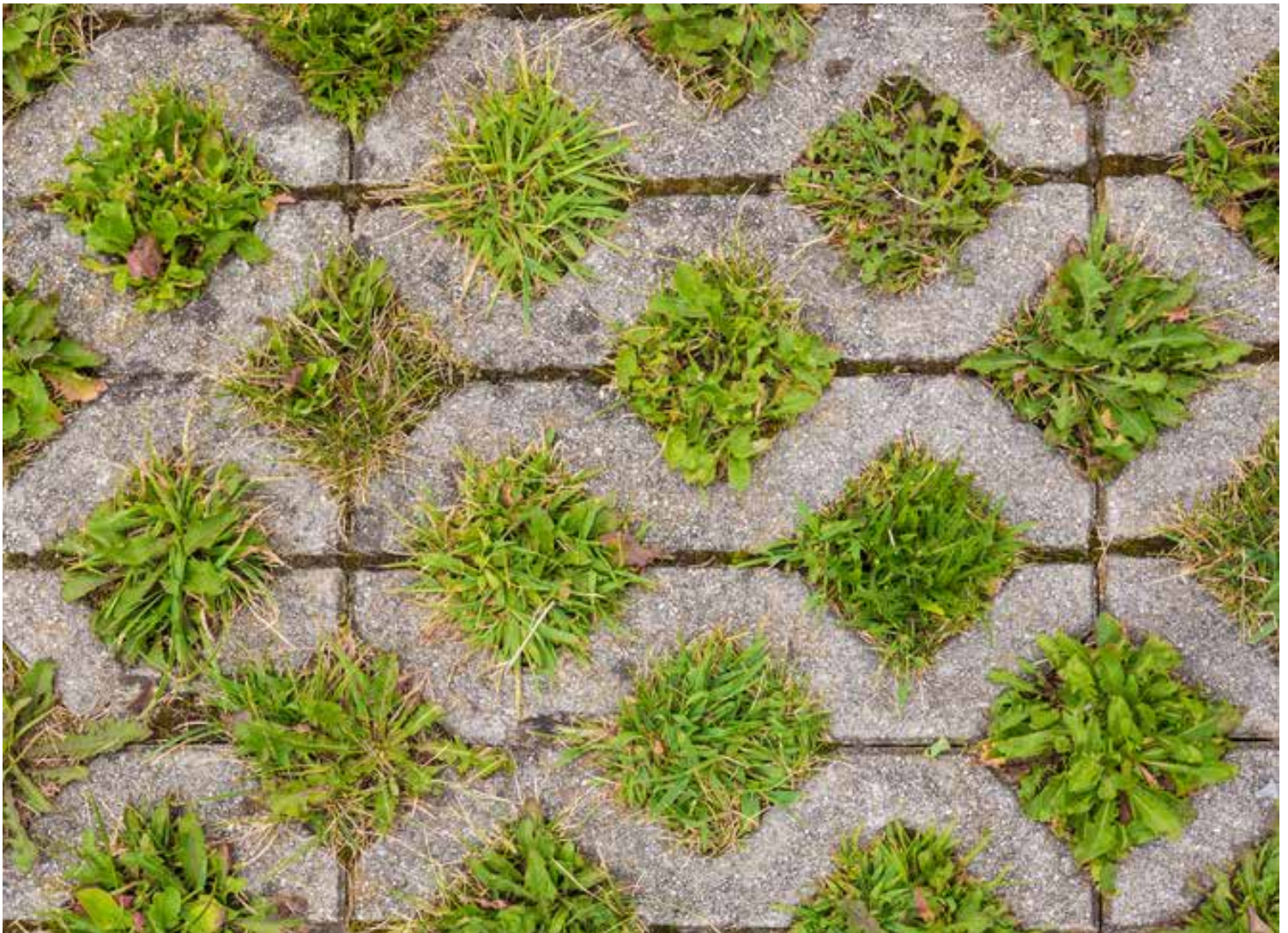
Figure 10. Permeable interlocking concrete pavers with oak leaves in gaps.
