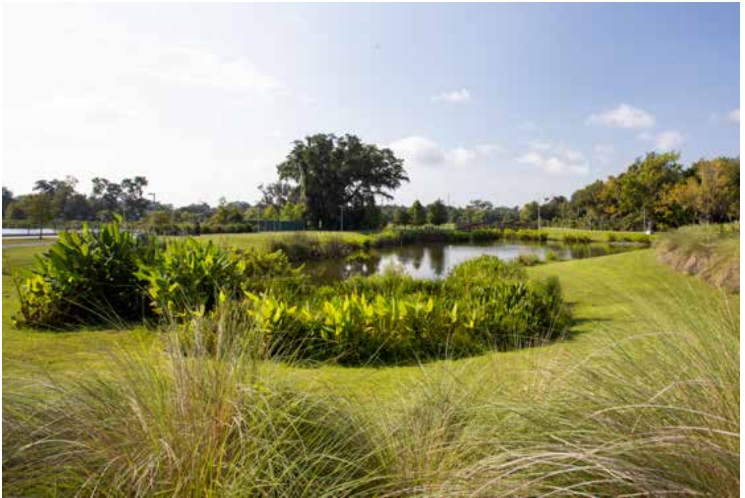
Figure 13. Stormwater pond with planted buffer at Depot Park in Gainesville, Florida.
