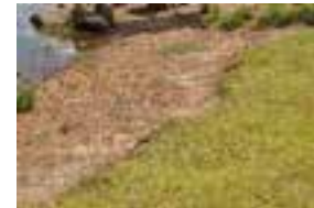
21 Erosion, plant, mulch
