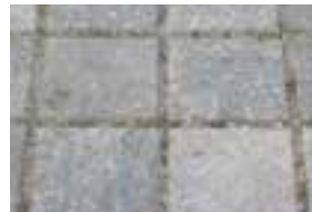
18 Sediment (poor)
