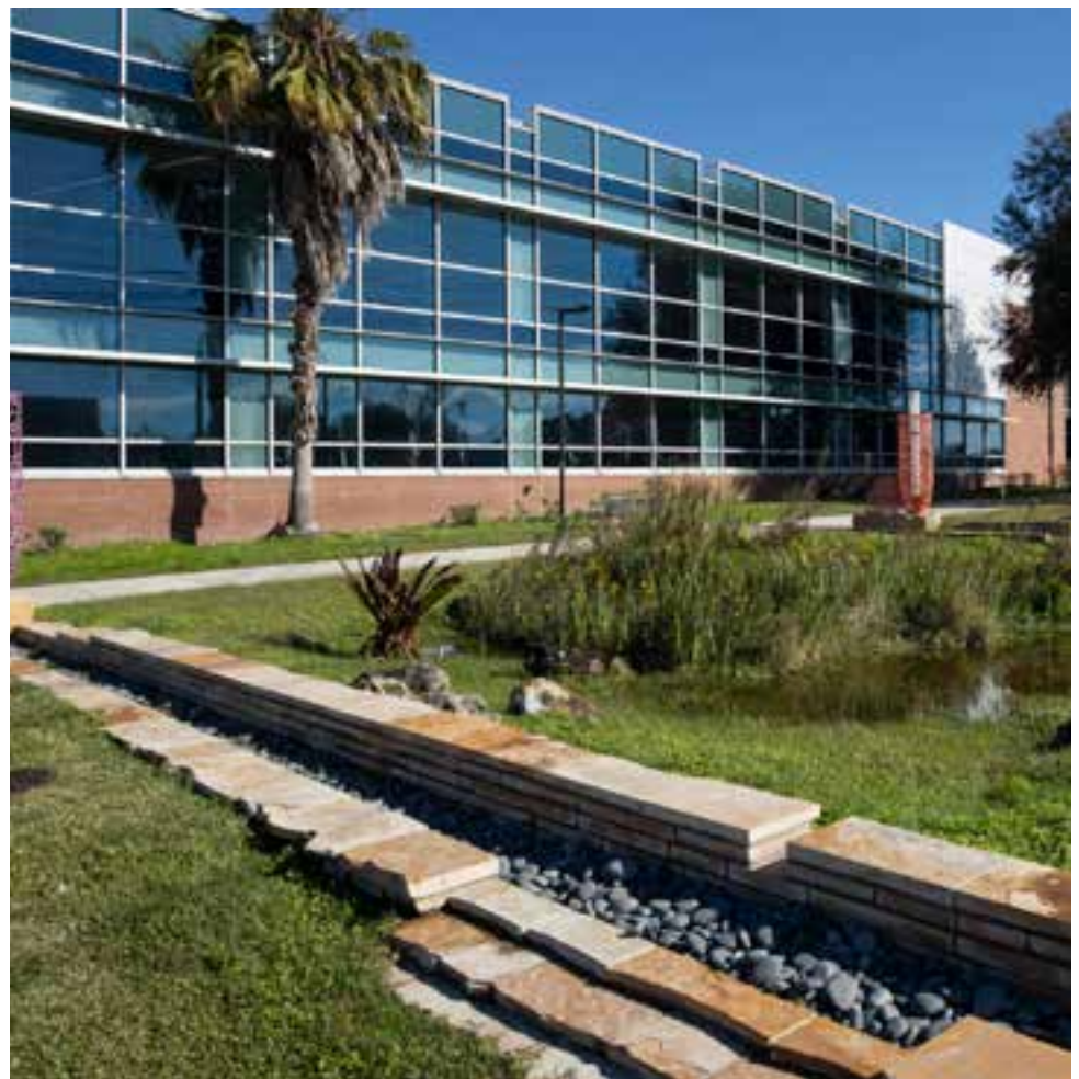
Figure 3. Extended ponding in bioretention on University of Florida campus.
